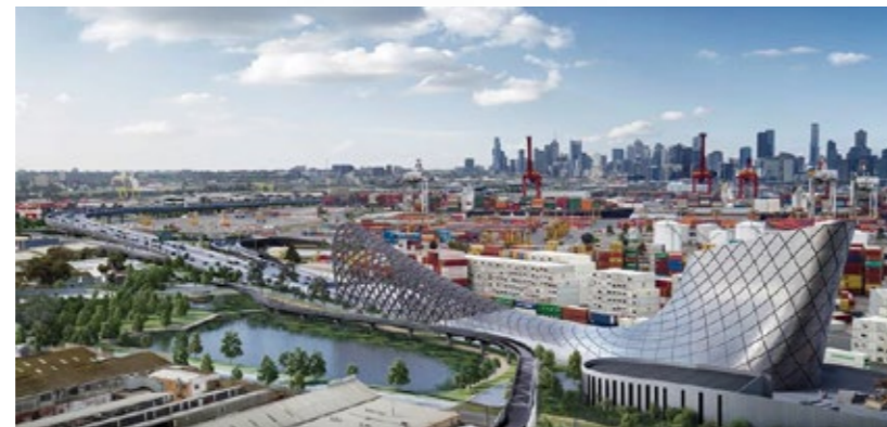
Westgate Tunnel \ A landmark timber gridshell over freeway tunnel portal celebrating Aboriginal heritage and culture.
