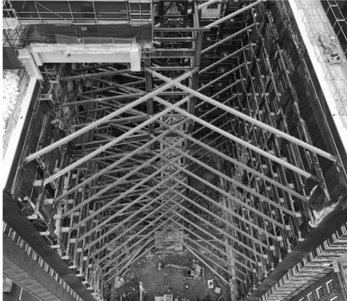
Shell House \ Shell House is one of the tallest retained heritage façades in the world and the temporary works one of the most complex projects of its kind
