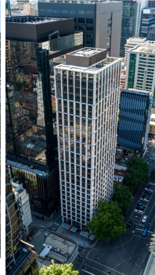
Iglu Russell Street \ A 28-storey student accommodation building in the heart of Melbourne. Photography by Kane Multimedia.
