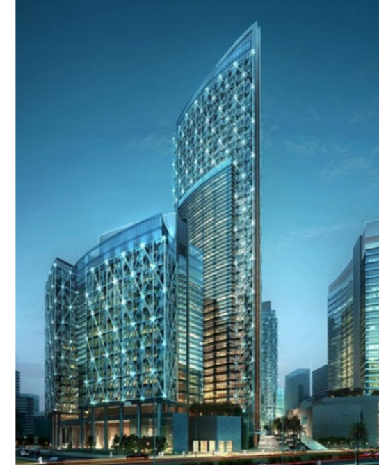
Barwa, Qatar \ A glass and travertine stone façade, where the glass is protected from the high heat exposure by metal screening inspired by the traditions of the precinct.
