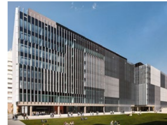
UNSW Material Science and Engineering Building \ 9-storey building enveloped by a high performance glass Façade with glass reinforced concrete masonry blades to provides solar shading
